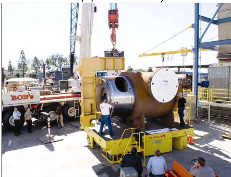
Figure 26. C85 Compressor Module Exchange
