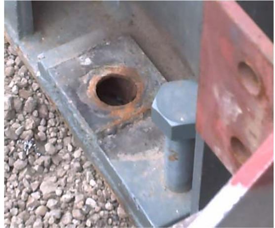
**Figure 3.2: Field Modified Avon Skid Anchor Bolt Hole**
