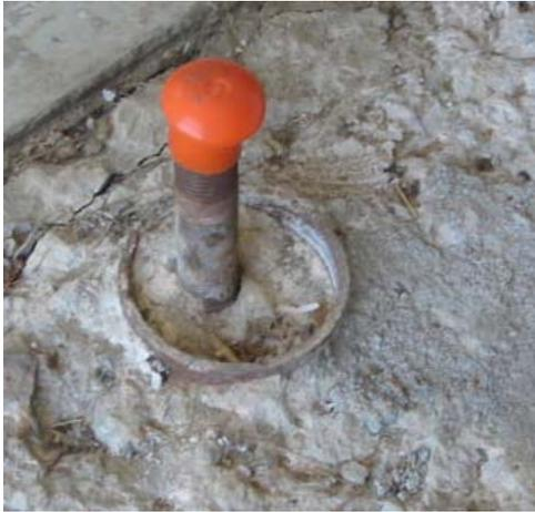
**Figure 3.1: Bright A1 Existing Anchor Bolt**
