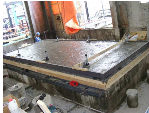
Figure 4 Foundations Re-leveled
