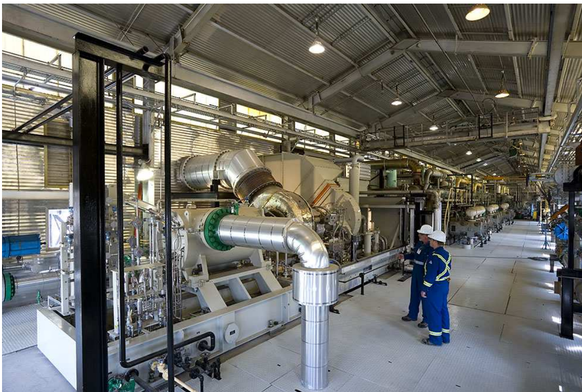
Figure 5 Turbine Final Installations
