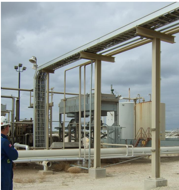
Newly installed cable raceways
