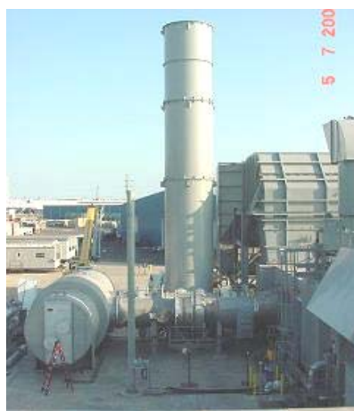
Fig. 19. LMS100™ Full Load Test In Houston
